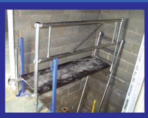
Stairsafe is the ideal width for stairwells, being 600mm wide it allows the correct amount of working space down the side of the platform for boarding, taping, plastering and decorating without there being a risk of falls.
