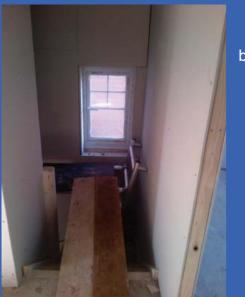
Where required an additional Stairsafe platform or scaffold boards (as shown) can be used to provide access onto the platform from the top of the stairs.
