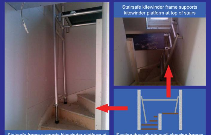
Stairsafe frame supports kitewinder platform at lower end of stairs
