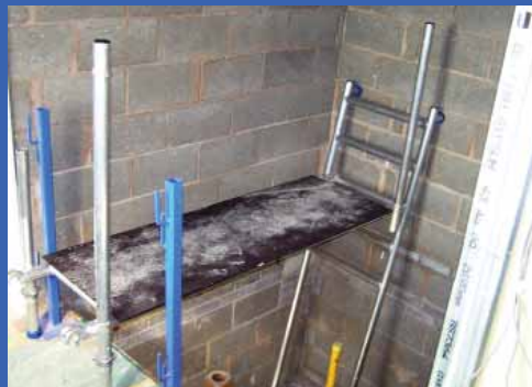
Guardrail posts fitted
