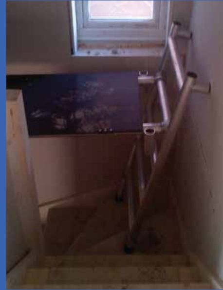
3 Position Kitewinder platform on frames
