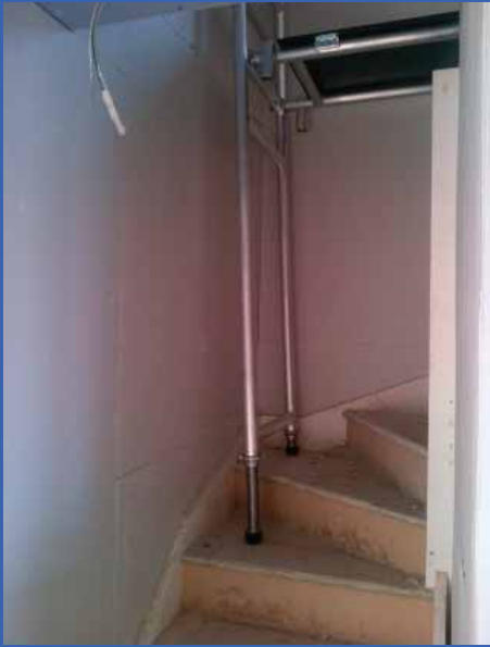
1. Position Stairsafe ladder frame at lower end of stairs
