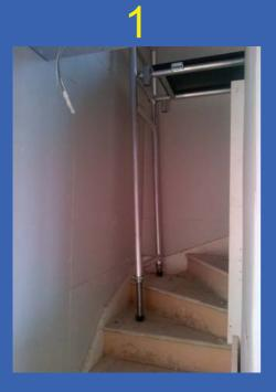
1. Position Stairsafe ladder frame at lower end of stairs
