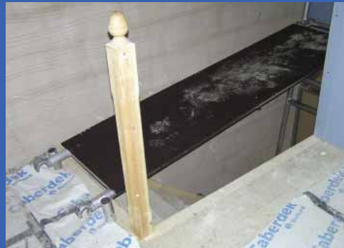
Platform in position
