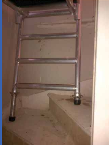
2 Position Stairsafe kitewinder frame at top of stairs
