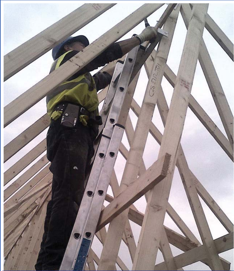
Ladder extends to correct level to suit truss height
