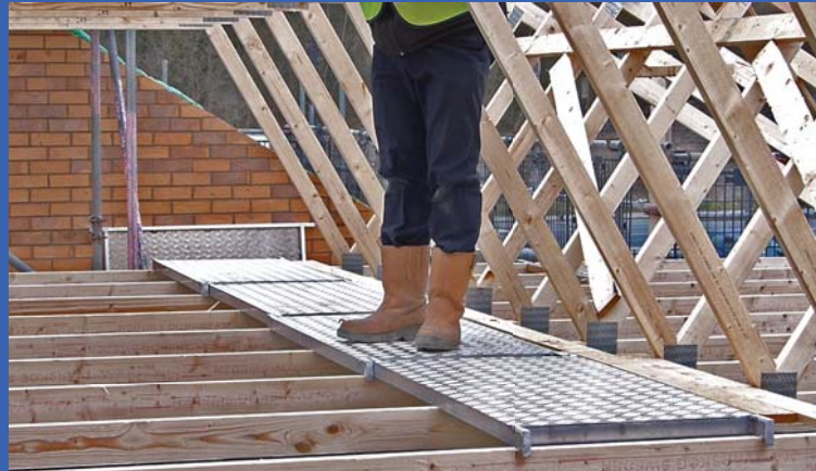
S.T.A. Panels can be used as a safe full length walkway
