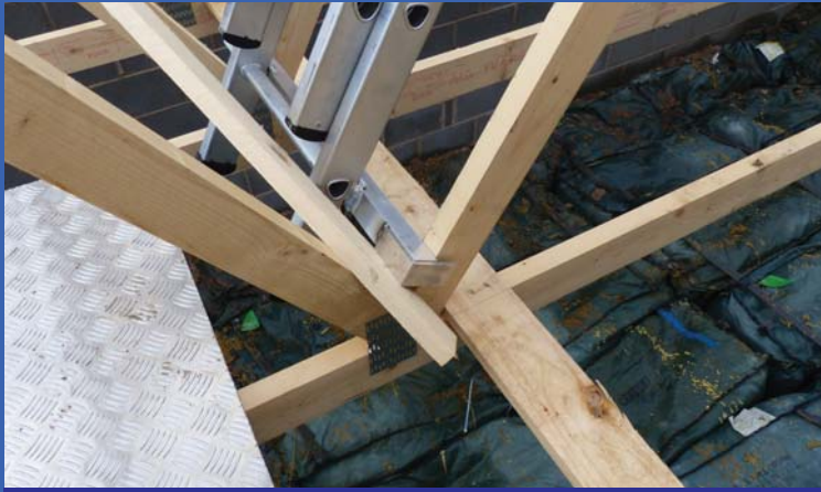
S.T.A. System in use with Soft Landing System
