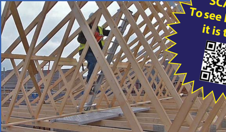
S.T.A. System in use with S.T.A. Panels with Soft Landing System below
