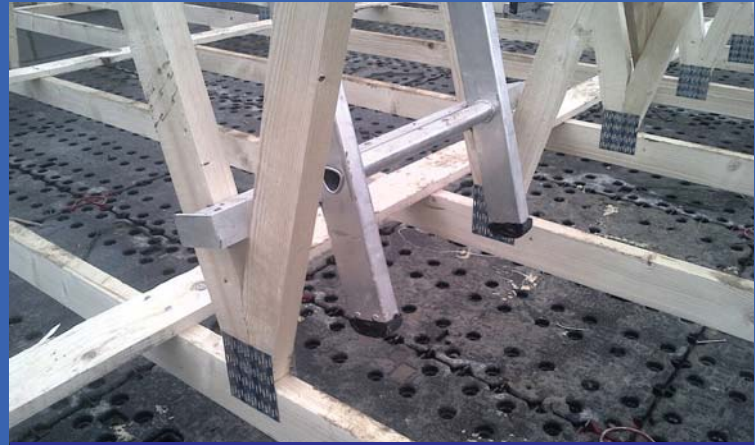
S.T.A. System in use with Decking System
