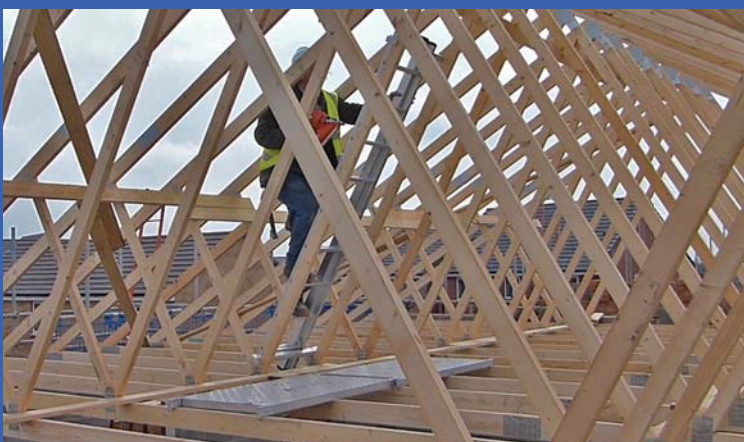
S.T.A. System in use with S.T.A. Panels with Soft Landing System below
