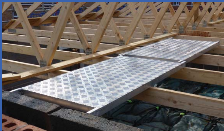
S.T.A. Panels provide safe access across roof trusses above Soft Landing System
